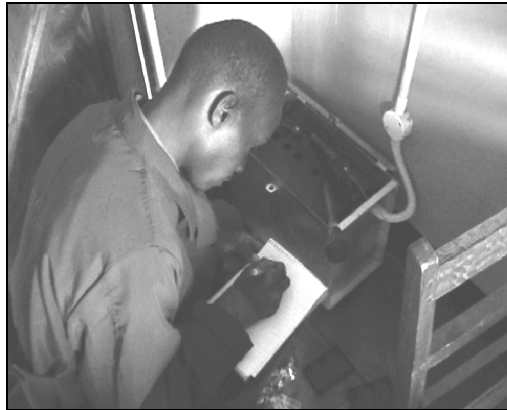
Figure 15: CHESCO technician checking the battery specific gravity
